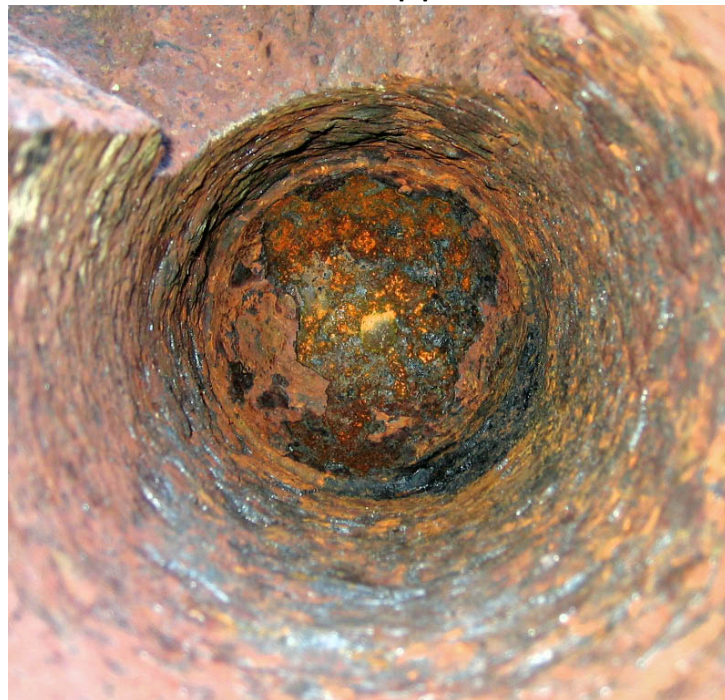
After water blasting and scraping bore to remove expanded rust
