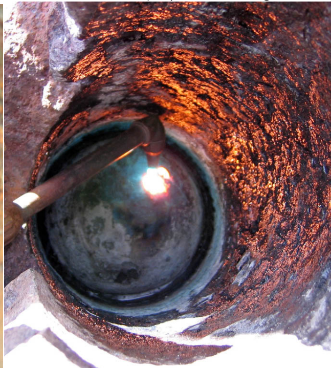
Flame heating the ball for over one hour.
