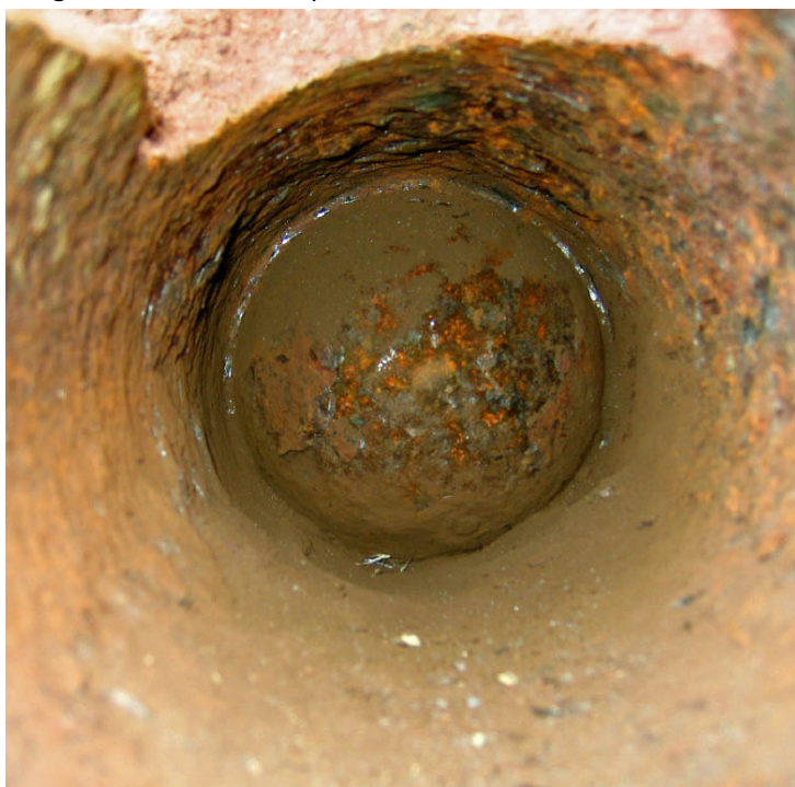
Rust dust from scraping between ball and bore.
